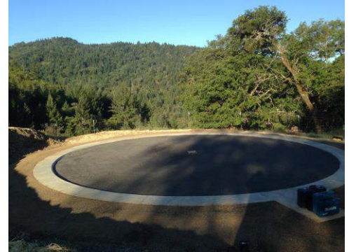
An example of a well-constructed ring beam foundation.
