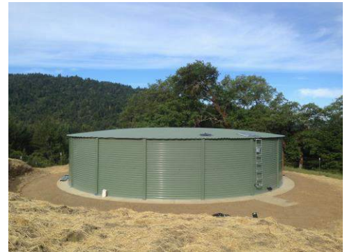
Completed tank, ready for anchoring.
